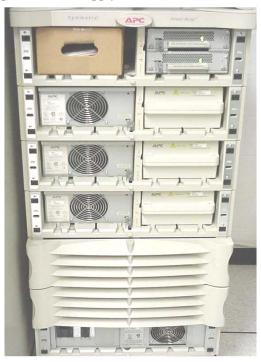
Until recently, loss of power to the Timer Room or Transmitter Room has resulted in Loran-C unavailability for the affected baseline. After evaluating and testing a number of uninterruptible power supplies during the past year, the Loran Support Unit (LSU) has installed APC Symmetra uninterruptible power "arrays", or supplies (UPS), at LORSTAs Jupiter, FL, Grangeville, LA, Carolina Beach, NC, and Malone, FL.
